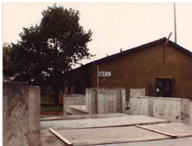
Building G-4 at Florennes
