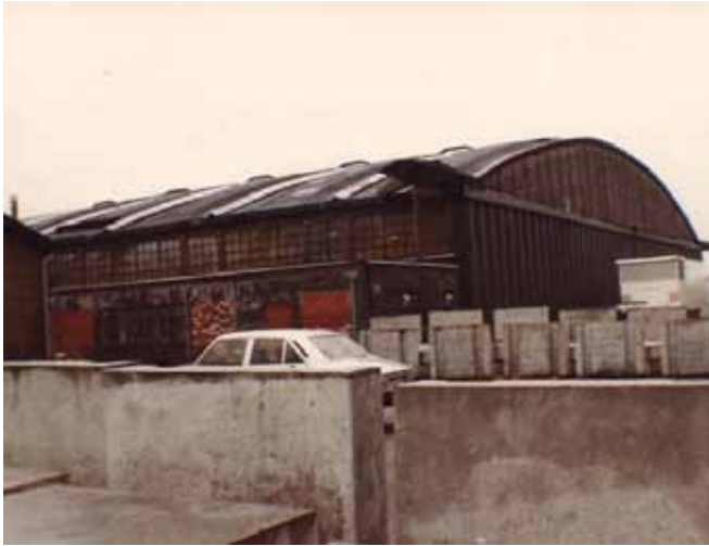
Building G-5 at Florennes
